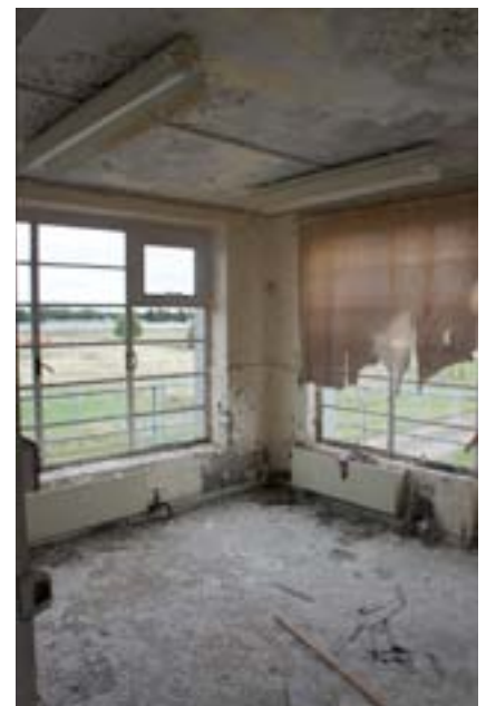
// Westcott Control Tower, 2012
